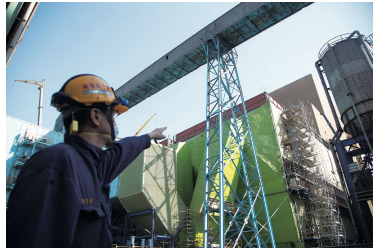
▼ Taichung Power Plant closed-trough conveyor belt system can reduce the escape of coal dust
