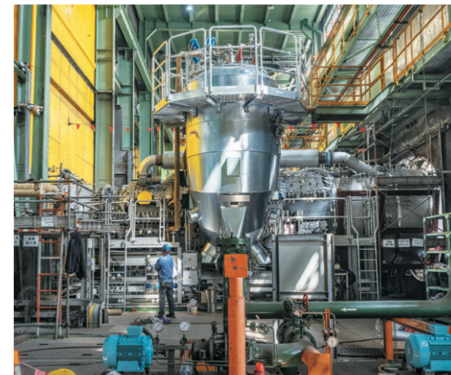
◀ Xinda Power Plant combined-cycle gas-fired units thermo-element upgrades
